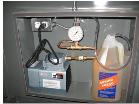
Odor Spray components Figure 4
